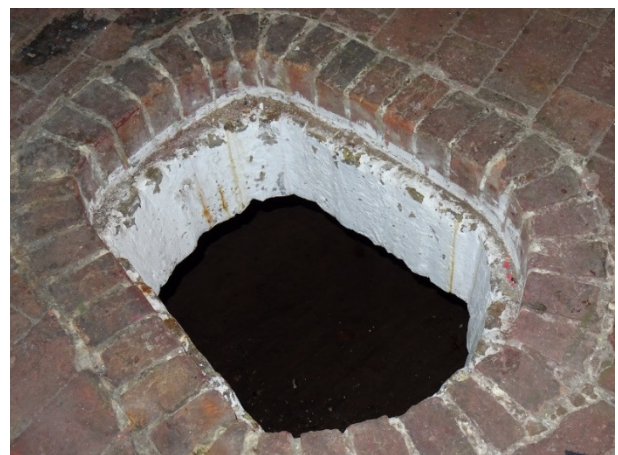
Western access into cistern, with trap hatch removed
