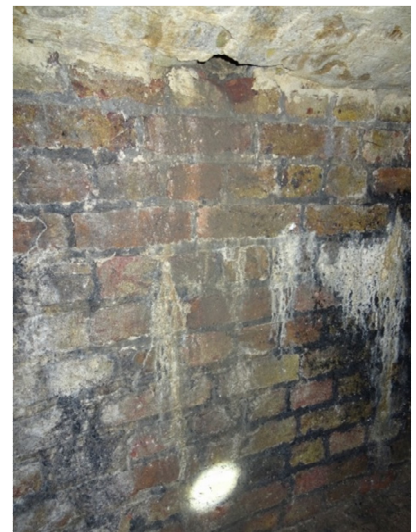
Point of potential water discharge from roof into cistern
