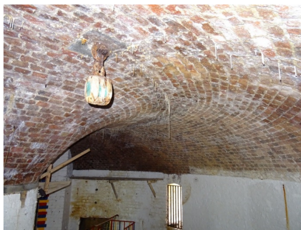
Roof vaulting with stalactites
