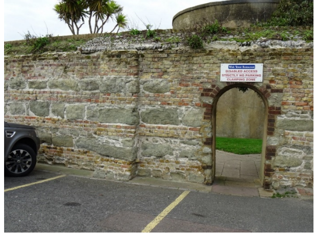
South (external) face of southern glacis wall
