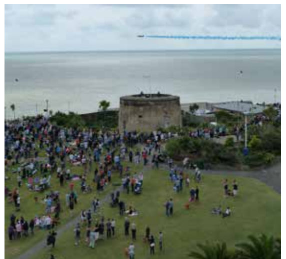
From top: The tower in its moat setting; visitors discussing construction of the interior of The Moat Wall; visitors enjoying Airbourne on the Slopes.
