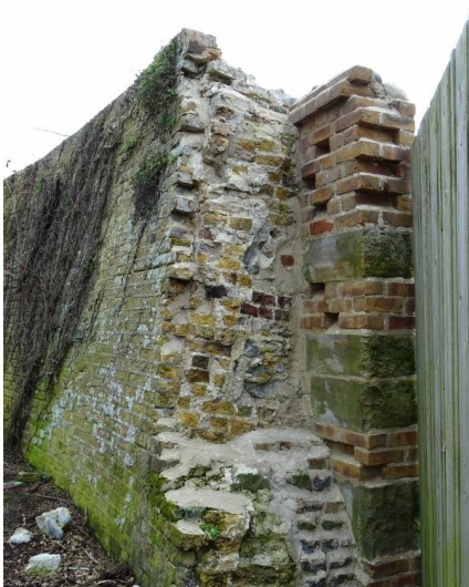
Exposed section through glacis wall showing solid bonding
