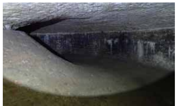
From top: exterior view of Wish Tower door; internal supporting pillar & arched roof; magazine/powder room; under-basement cistern with inverted arch.
