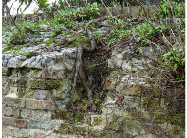
Cobbled capping to glacis wall
