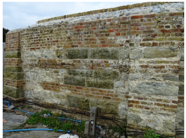
Previously repaired section of glacis wall at south-west end
