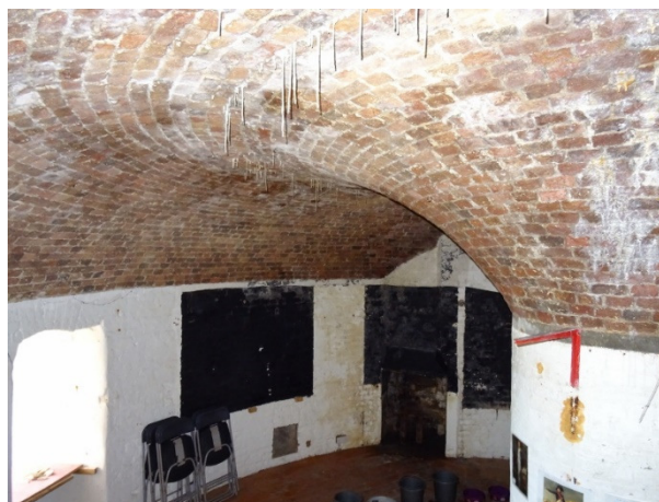
Roof vaulting to accommodation level towards the east. Note stalactites
