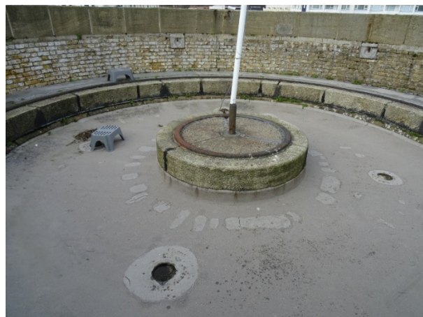
General view of gun platform roof
