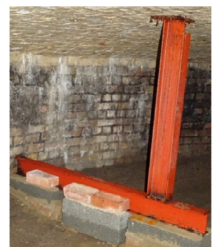
Modern steel strutting
