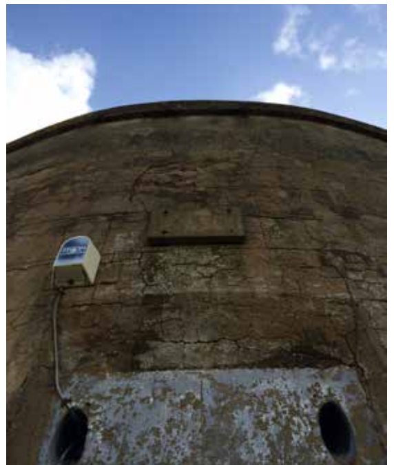
From top: internal view showing double-height space; vaulted stairs to roof prior to clearance work; detail over front door showing drawbridge rope holes.
