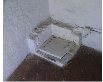
Eastern sump into cistern,
